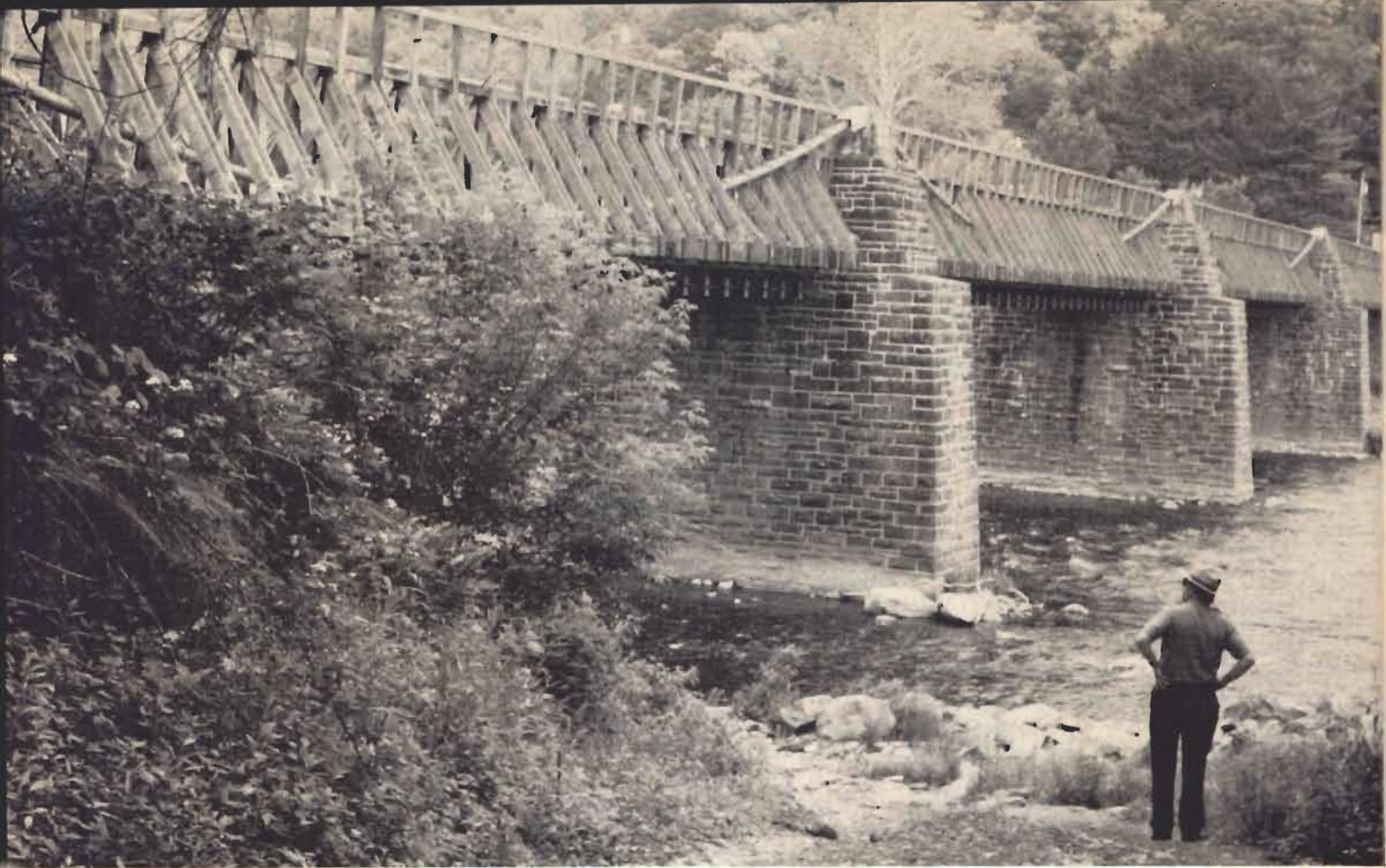
The Roebling Bridge, the oldest standing suspension bridge in the United States and a national landmark constructed by the designer of the Brooklyn (New York) Bridge, spans the Delaware River at Lackawaxen, Pike County. The structure was built in 1848 as an aqueduct to carry the Delaware & Hudson Canal over the river.
