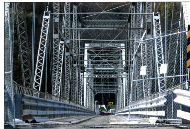
Struts and trusses.
