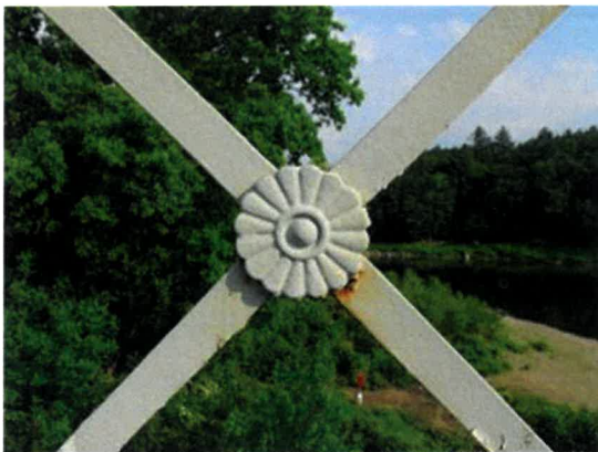
Flower motifs on bridge railings.
