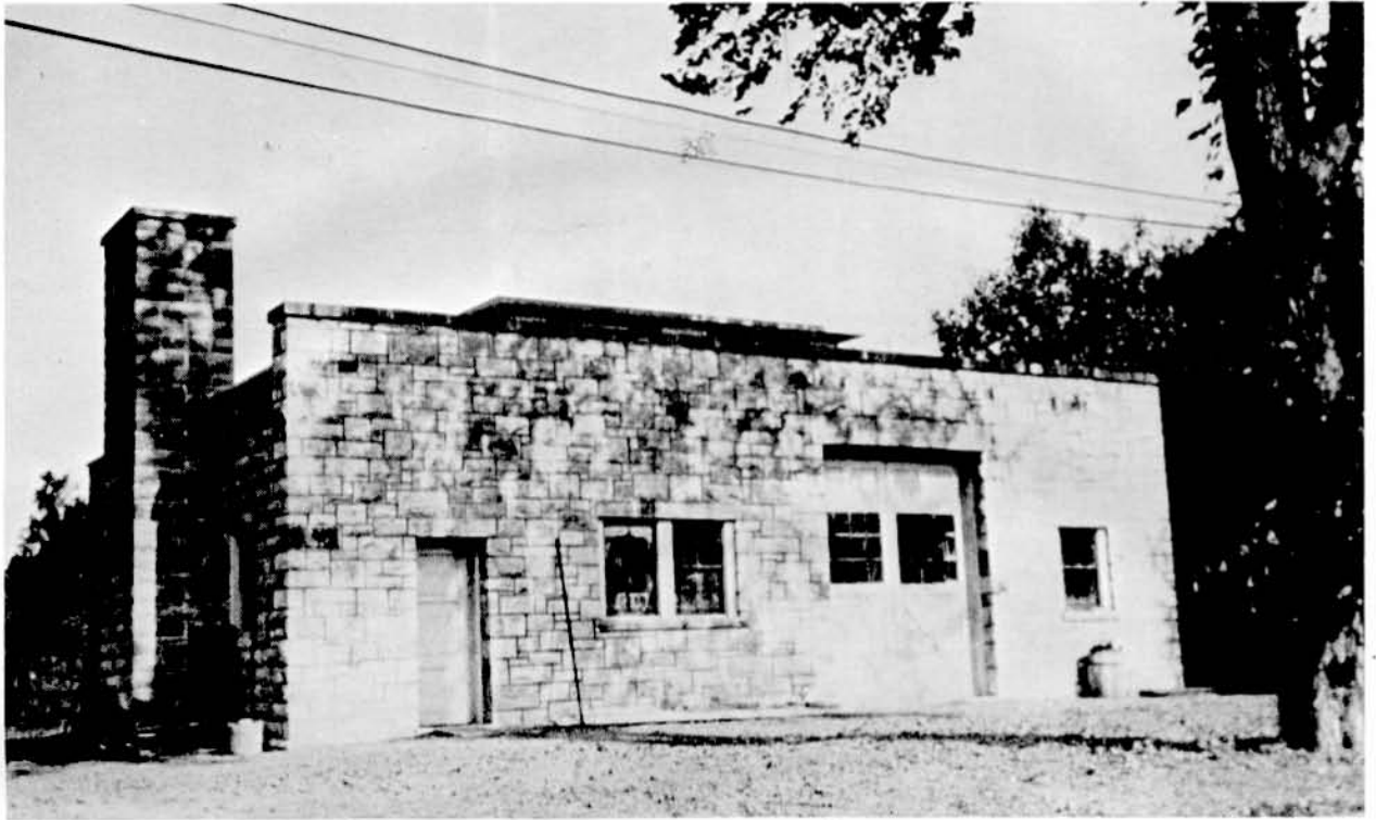
Second Blacksmith Shop
