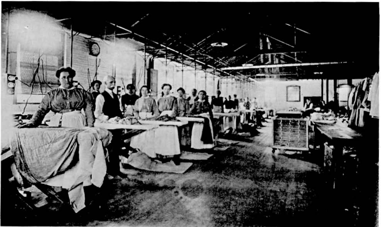
Second Floor of Laundry Built 1886
