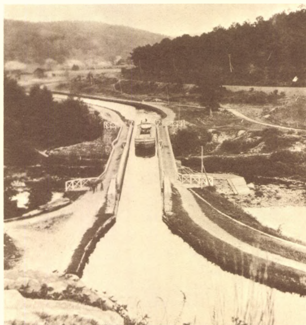
FIGURE 30.—One of the last boats through the canal crossing the Lackawaxen Aqueduct, about 1898, moving light toward Honesdale. On the Delaware and Lackawaxen aqueducts the towpath was widened around the midstream towers to provide a constant width; the path on the berm side, however, used mainly by common foot traffic, was not widened. (Photograph courtesy of Delaware & Hudson Railway Company.)
