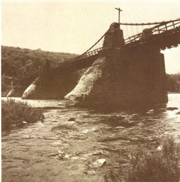
FIGURES 51 and 52.—The contrasting massiveness of masonry piers and lightness of wire cables, so much the measure of the suspension bridge and so often extolled by poet and painter in the Brooklyn Bridge, is as fully marked at the aqueduct.
