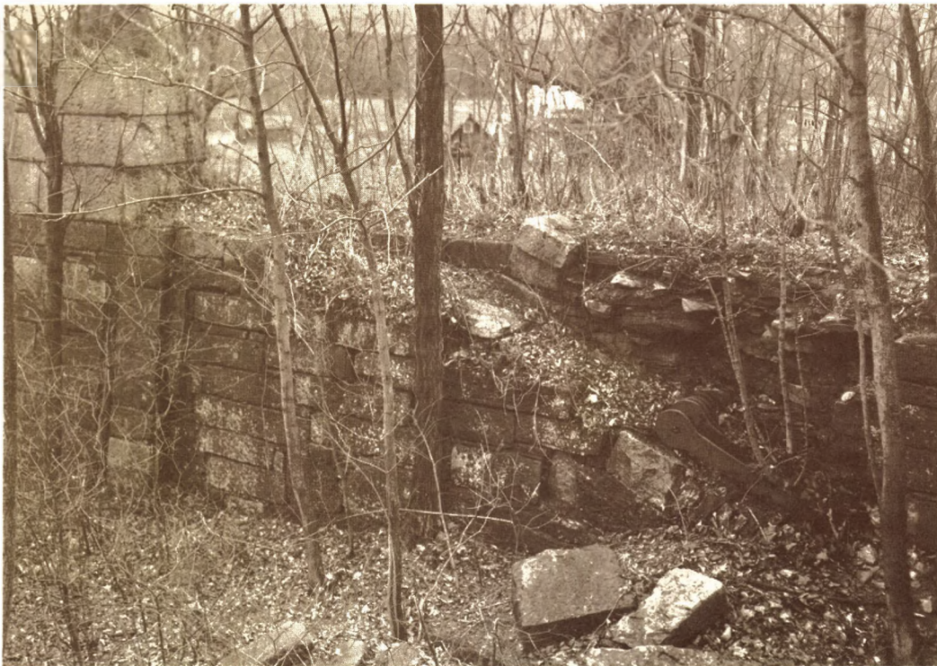
FIGURES 38 and 39.—The masonry of both Neversink Aqueduct abutments survives, but all the upper sections of the anchor bars are gone. Just upstream on both sides of the Neversink are fragmentary remains of the predecessor two-span timber-truss aqueduct. As at High Falls, the canal was slightly realigned during the enlargement to permit construction of the new aqueduct without disrupting service on the old. On both of the later structures, the abutment wing walls are straight, meeting the face at an angle, unlike the earlier Delaware and Lackawaxen spans where the surfaces meet in a curve. (Historic American Engineering Record and the Smithsonian Institution.)
