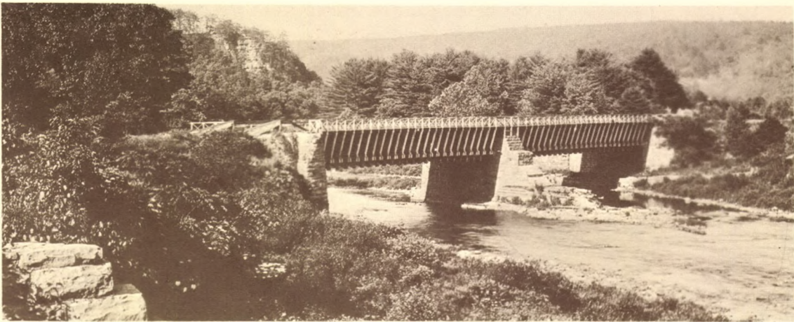
FIGURE 31.—The Lackawaxen Aqueduct, looking northeast toward the Delaware. As at Pittsburgh, Roebling arranged the floor beams and side struts of the Delaware & Hudson aqueduct trunks into simple trusses that both supported the overhanging towpaths and resisted the side pressure of the water on the trunk walls. (Photograph courtesy of Delaware & Hudson Railway Company.)
