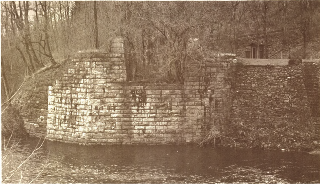
FIGURES 38 and 39.—The masonry of both Neversink Aqueduct abutments survives, but all the upper sections of the anchor bars are gone. Just upstream on both sides of the Neversink are fragmentary remains of the predecessor two-span timber-truss aqueduct. As at High Falls, the canal was slightly realigned during the enlargement to permit construction of the new aqueduct without disrupting service on the old. On both of the later structures, the abutment wing walls are straight, meeting the face at an angle, unlike the earlier Delaware and Lackawaxen spans where the surfaces meet in a curve. (Historic American Engineering Record and the Smithsonian Institution.)
