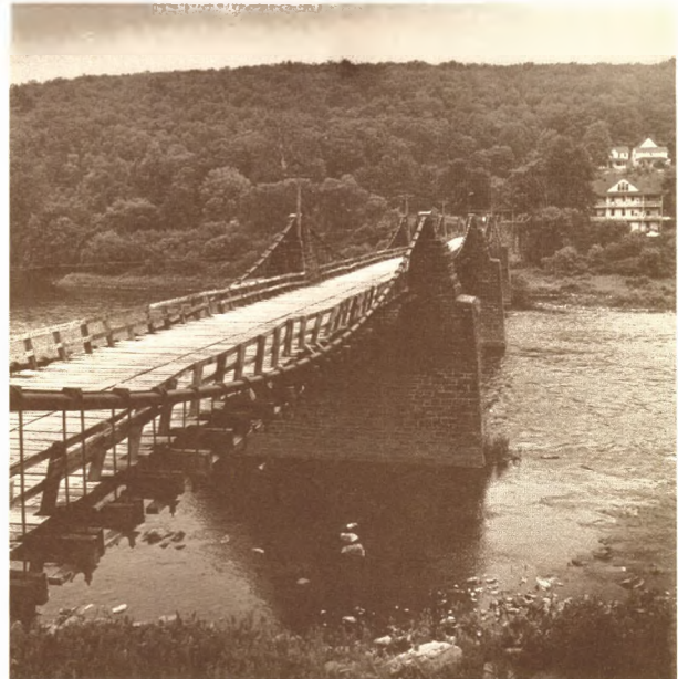
FIGURES 51 and 52.—The contrasting massiveness of masonry piers and lightness of wire cables, so much the measure of the suspension bridge and so often extolled by poet and painter in the Brooklyn Bridge, is as fully marked at the aqueduct.
