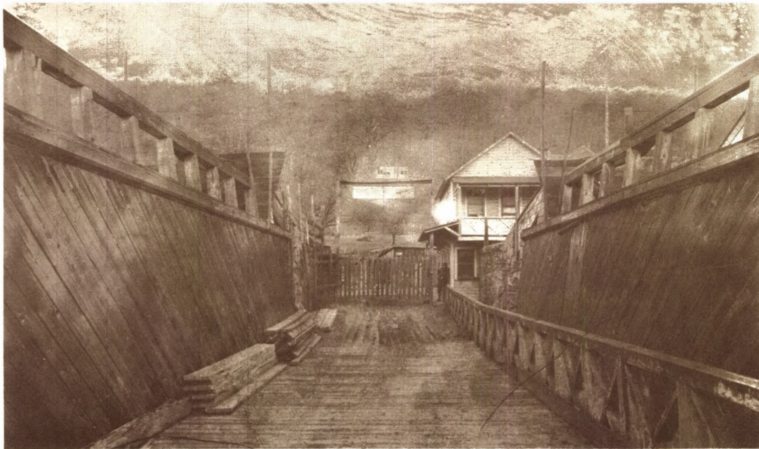
FIGURE 41.—Interior of the Delaware Aqueduct trunk after conversion to a toll bridge, about 1900. (Photograph courtesy of the Delaware & Hudson Railway Company).
