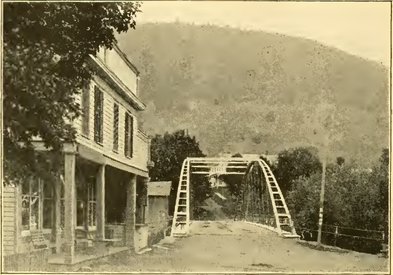
THE BRIDGE AT LEXINGTON.
